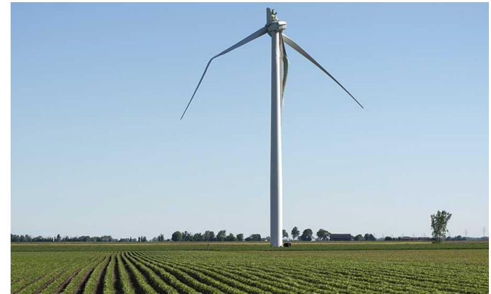
Blade failure
